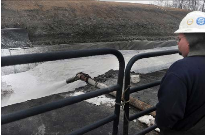
Harold Westfall of Barber County, W.Va., watches as foam pumps out of the ground and into a containment area at a Rice Energy Marcellus Shale drilling rig in Lone Pine, Washington County. Michael Henninger/Post-Gazette
